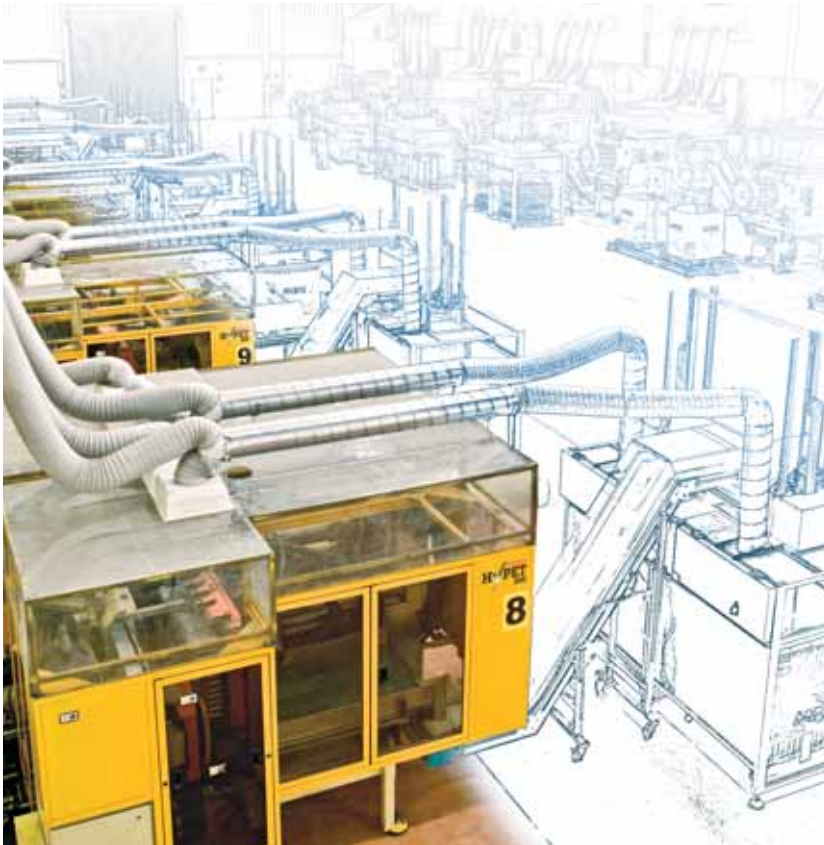
Husky experts conduct detailed assessments of customer facilities to identify areas of improvement.
